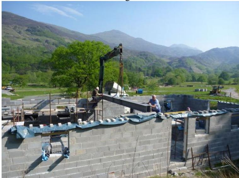
**Figure 3. Installation of Roofing Beam**
